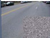
Has the same appearance as hot mix asphalt, but it is more porous resulting in better traction numbers.
