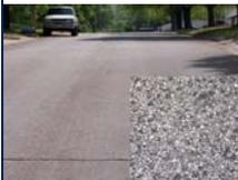
After oil has cured (2-4 hours depending on temperature), it has the appearance of new asphalt.
